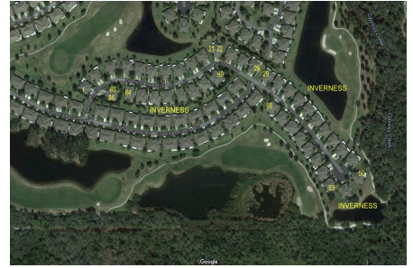
Built in 2003 - 86 units - 1 floor
