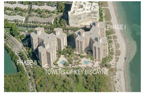
Built in 1972 - 262 units (538 with phase 2)- 16 floors
