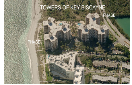
Built in 1972 - 276 units (538 with Phase 1) - 16 floors
