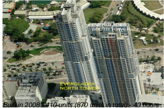
Built in 2008 - 410 units (870 units in total) - 49 floors
