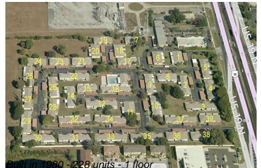
Building # 160 - 228 units - 1 floor
